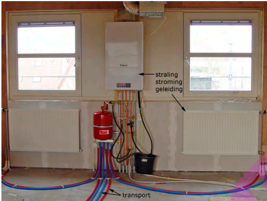
Warmte-afgifte via transportmedium water
